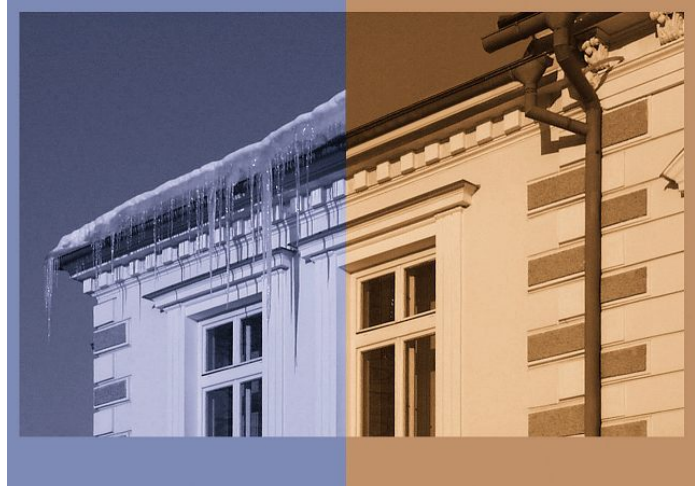
Without Flexel heating cable With Flexel heating cable
